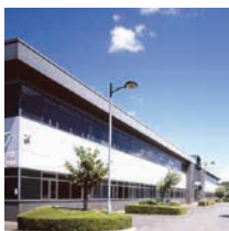
Redhill Data Centre, Redhill, Great Britain.
