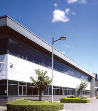
Redhill Data Centre, Redhill, Great Britain.
