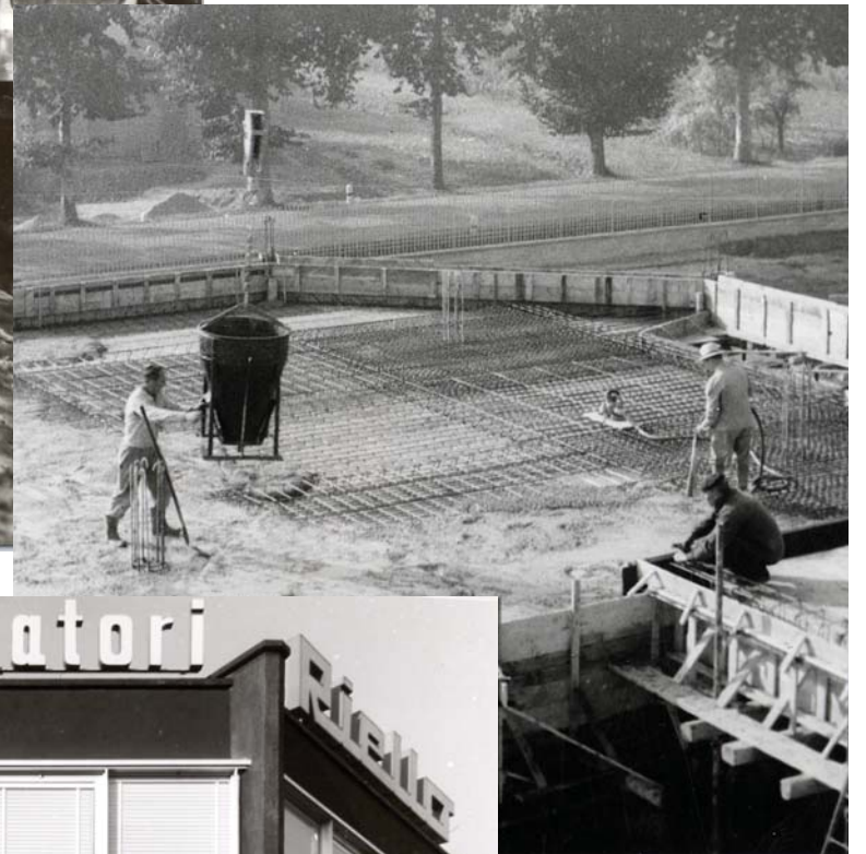
Below: the concrete casting for the Ottagono, the headquarters office.
