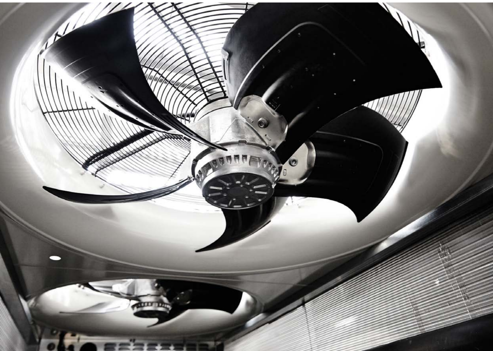
Latest generation fans on an Aermec chiller
